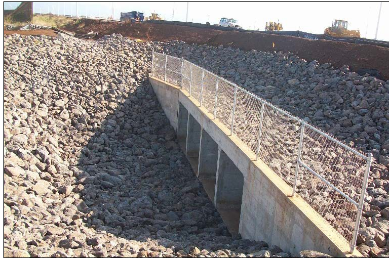
Image Source: State of Hawaii Department of Transportation, Highways Division, Construction Best Management Practices Field Manual , 2021.
